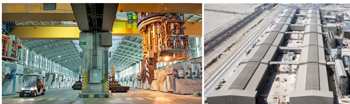
Figure 8. Qatalum smelter potroom with two rows of HAL 250 cells (left) [7] and the smelter with two potlines (right) [8].
